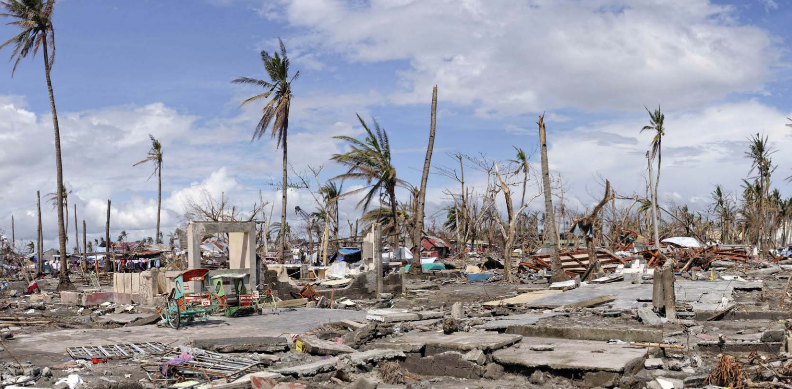
Damage from Typhoon Haiyan (Yolanda) that struck Tacloban in the Philippines on November 8, 2013. It was one of the strongest tropical cyclones ever recorded and impacted large portions of Southeast Asia, in particular the Philippines where it killed at least 6,300 people, making it the deadliest Philippine typhoon on record. Photo: © ILO / Marcel Crozet
